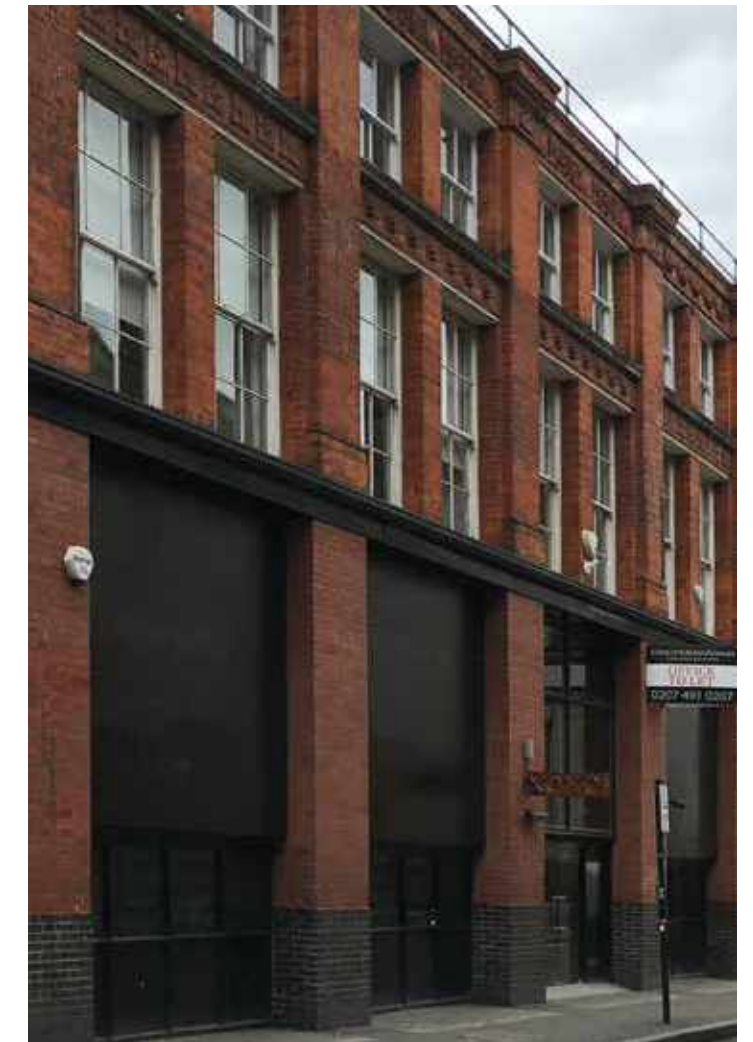
Warehouse double height bays
