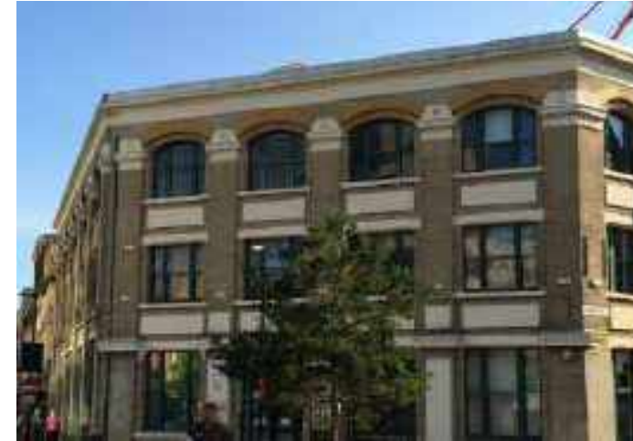
4 View of Victoria House from Leonard Circus, building of townscape merit
