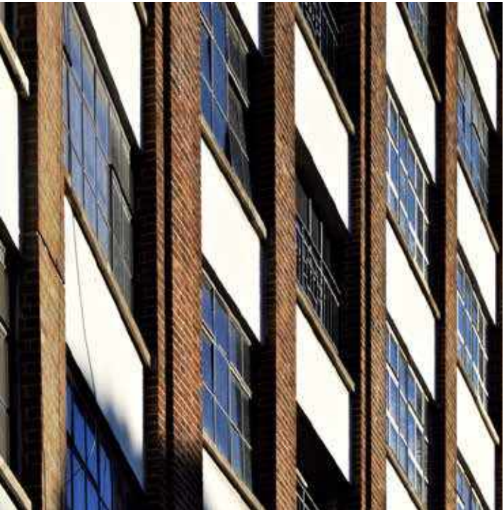
Double brick reveal detail, Tea Building
