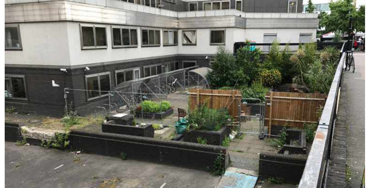
View of the sunken courtyard created by the demolition of part of the 50's building
